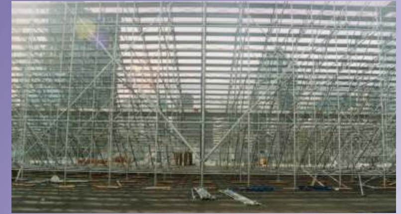
Typical rear view of Grandstands
